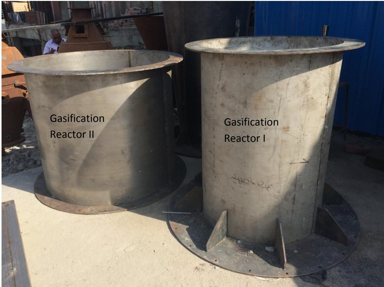
Figure 10: A view of the gasification reactors during the manufacturing process
